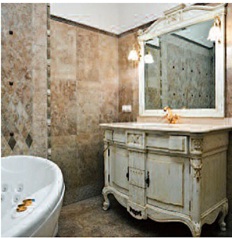
Bathroom Remodeling Tile Install - Repair
