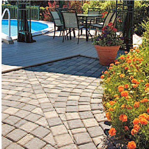
Paving Stone Install - Repair
